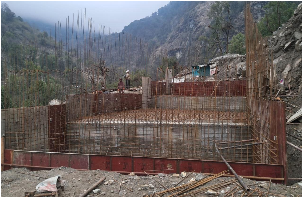
Figure 9: Formwork in AB 12
