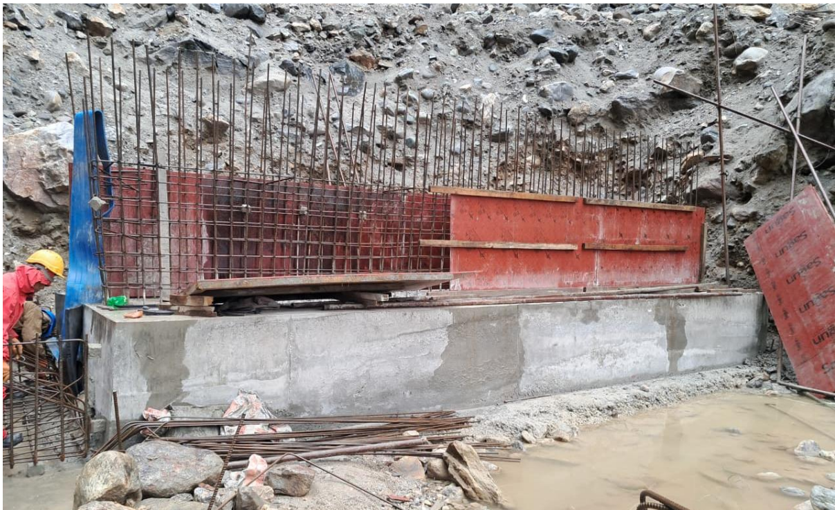
Figure 2: Rebar and formworks in Undersluice u/s cutoff in Headworks
