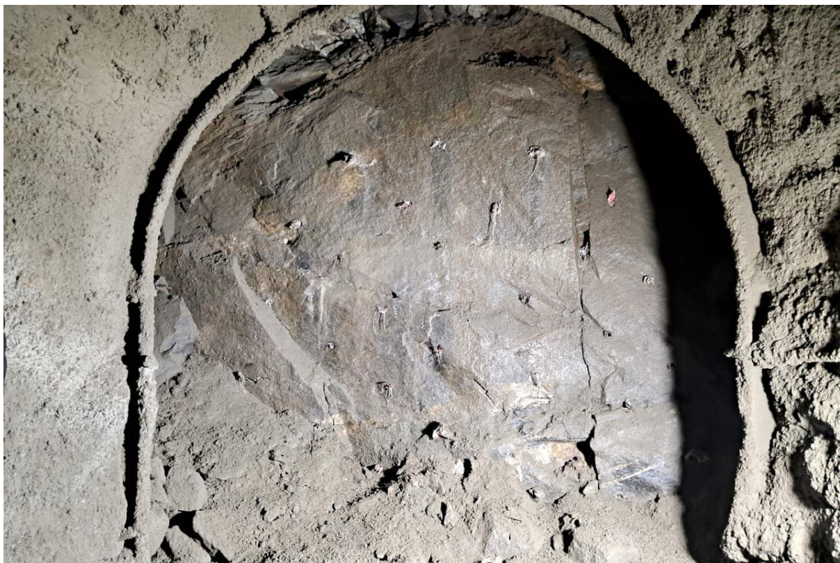
Figure 6: Inlet tunnel face at ch 0+017.40m
