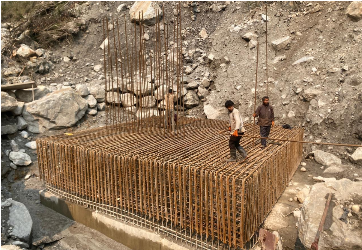
Figure 11: Rebar work in Bridge left abutment
