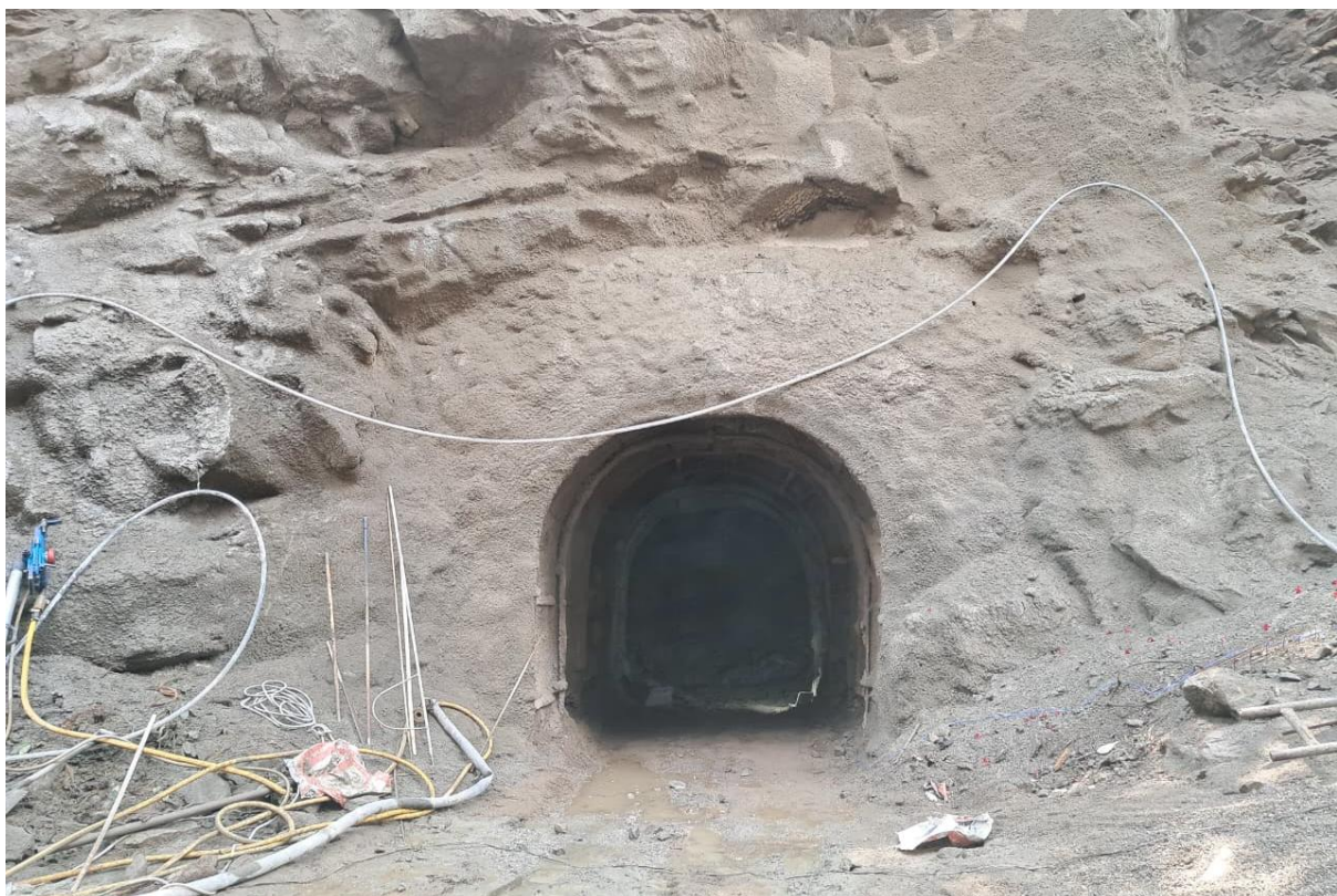
Figure 4: Shotcreting in Inlet Portal
