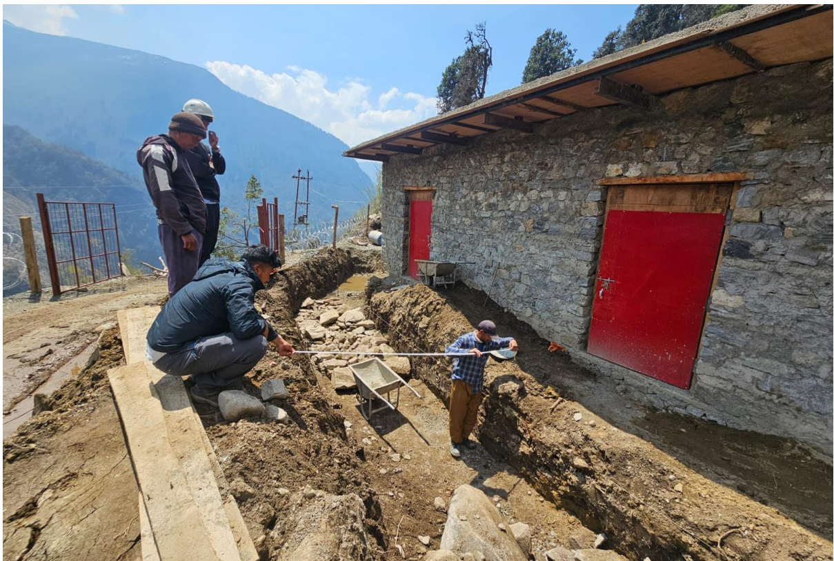
Figure 16: Foundation of Bunker traverse wall
