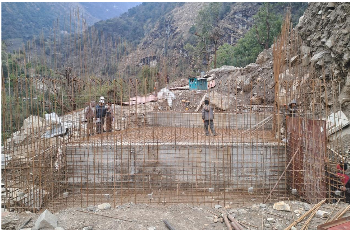
Figure 8: Rebar work in AB 12
