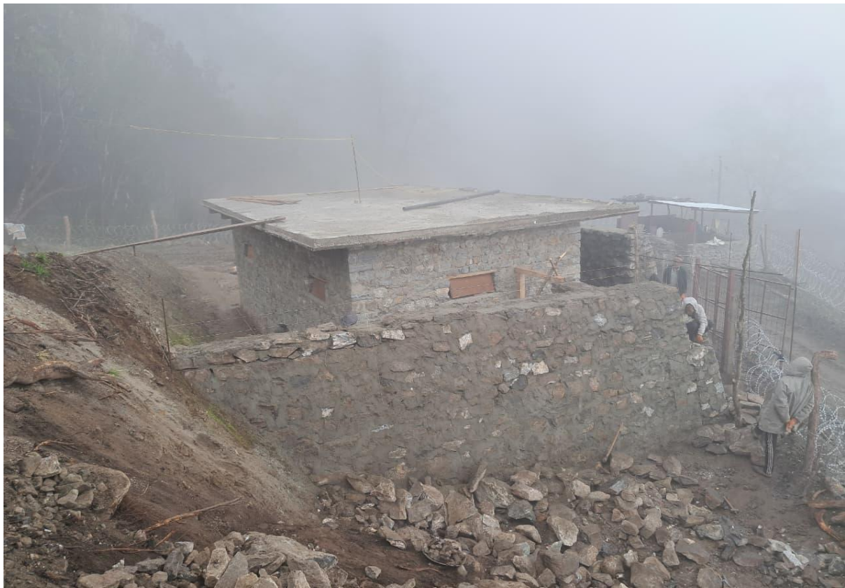
Figure 17: Traverse wall of Emulsion bunker
