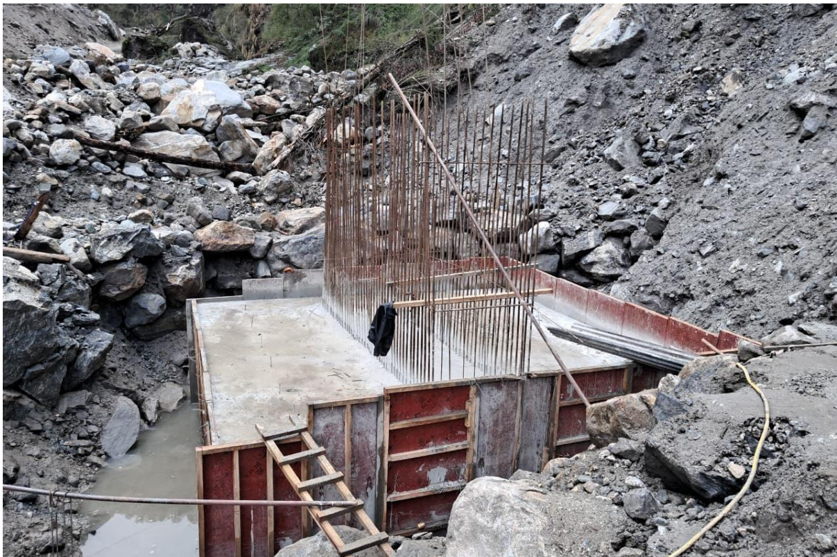
Figure 12: Base concreting in Bridge left abutment
