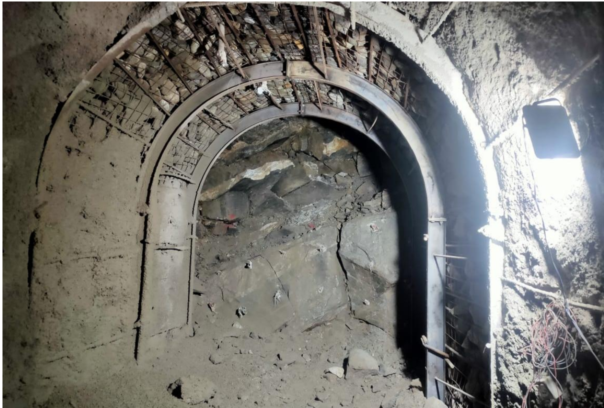
Figure 5: Inlet tunnel face at ch 0+010.20m
