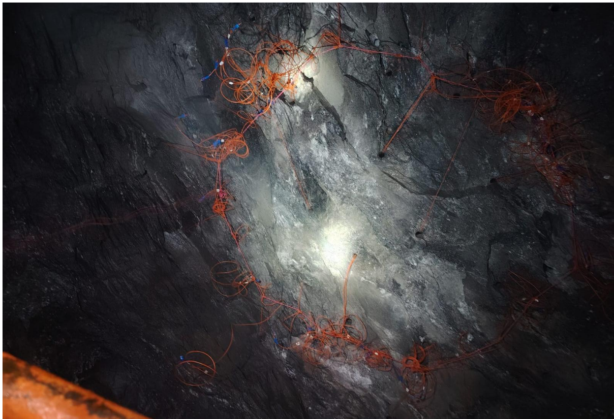
Figure 7: Preparation for blasting in Vertical Shaft
