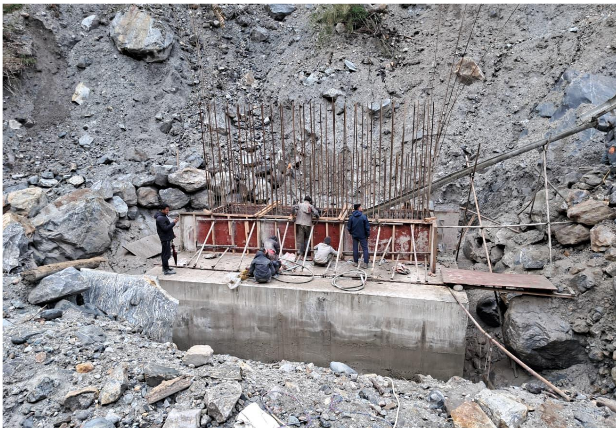
Figure 13: Preparation for first lift of stem wall of Bridge left abutment
