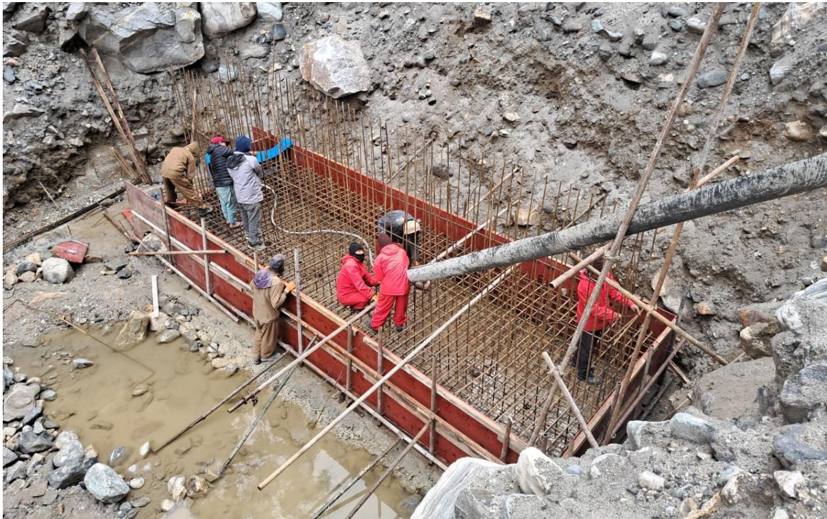
Figure 1: Preparation for concreting in Undersluice u/s cutoff
